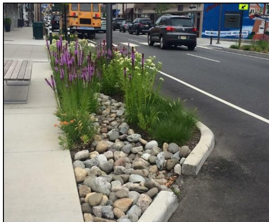
Figure 2. Rain gardens and curb bump-outs are often used together in urban settings. The curb bump-out leaves enough space for a rain garden while also improving pedestrian safety at busy street crossings.
