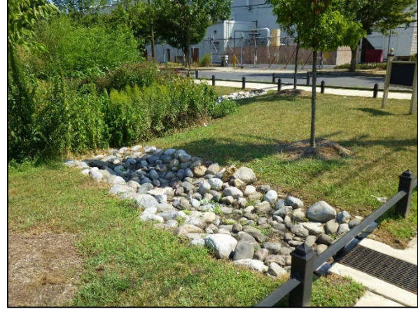
Figure 6. Riprap-lined inlet channel to a bioretention area in the Waterfront South rain gardens.
